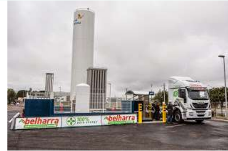
Station GNL/C de Castets
